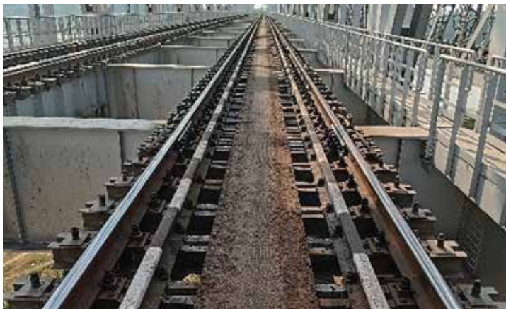
Transformation at Sampriti Setu, Eastern Railway – Howrah Division, West Bengal : From Corroded Mild Steel to Resilient Stainless Steel Chequered Plates - A Bridge to Durability and Reliability
