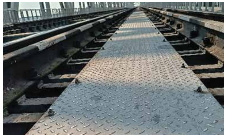
Transformation at Sampriti Setu, Eastern Railway – Howrah Division, West Bengal : From Corroded Mild Steel to Resilient Stainless Steel Chequered Plates - A Bridge to Durability and Reliability
