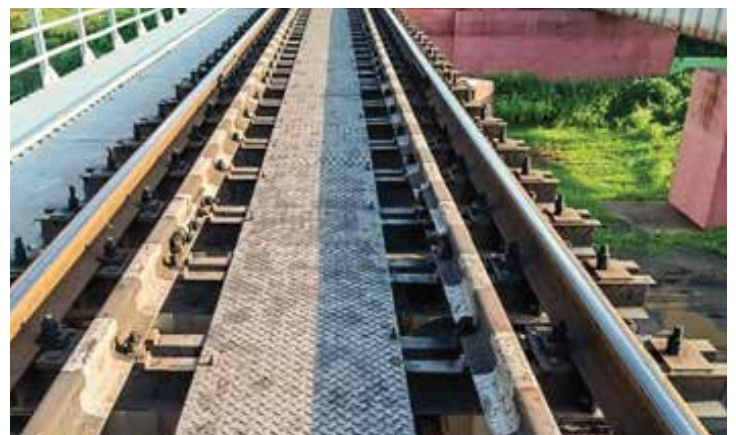
Revitalizing Nalhati Bridge, Eastern Railway – Howrah Division, West Bengal : Evolution from Corrosion-Prone Mild Steel to Enduring Stainless Steel Chequered Plates - Ensuring Longevity and Strength.
