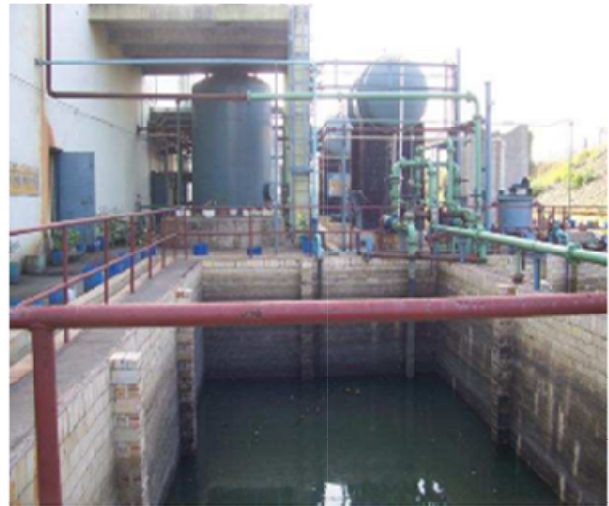
Neutralization Pit at DM Plant, CPP
