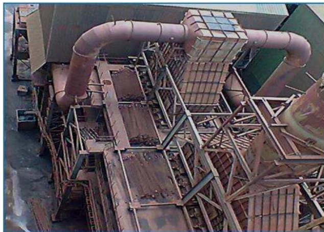
Pulsejet bag house used to control dust emission
