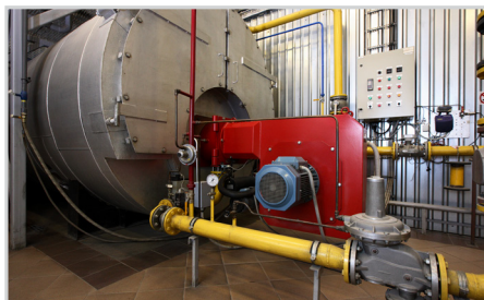
Oil Burner components
