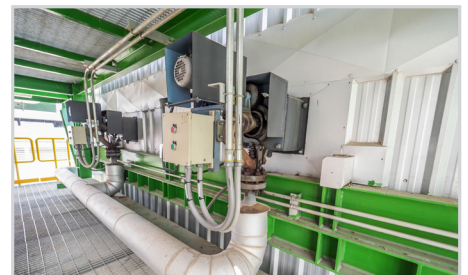
Soot blower systems
