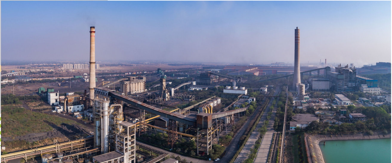
Aerial view of Jindal Stainless Limited, Jaipur
