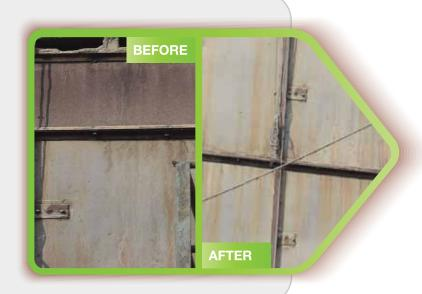
The picture shows Mild Steel getting corroded, while for the same period of exposure Stainless Steel lasts longer without any sign of corrosion
