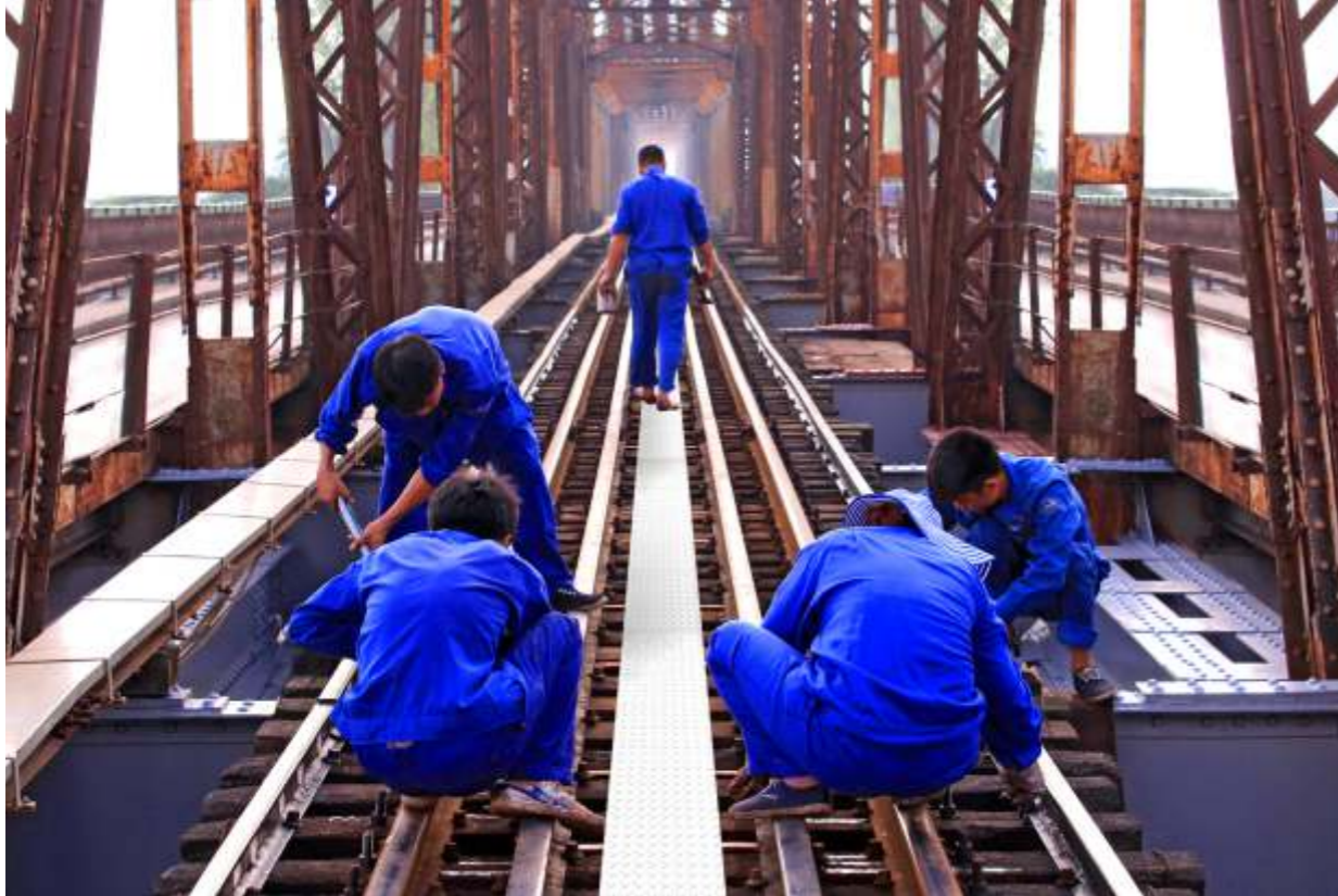
Railway Bridge Pathway: Ensuring safety & convenience during maintenance and inspections.
